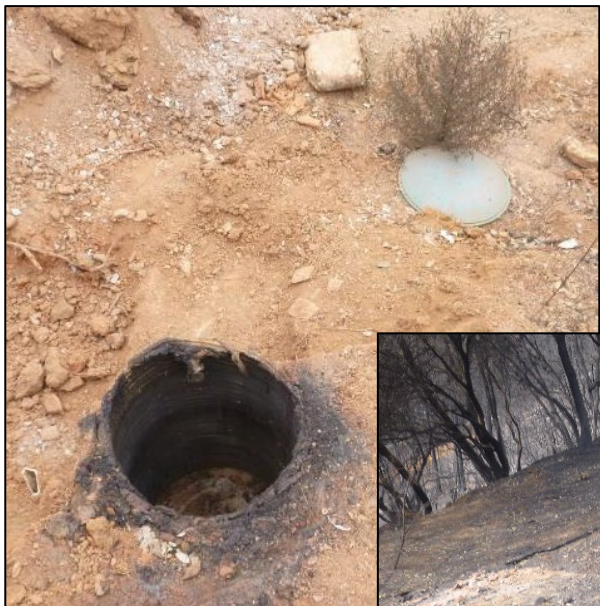
Open unmarked septic tanks after fire damage
