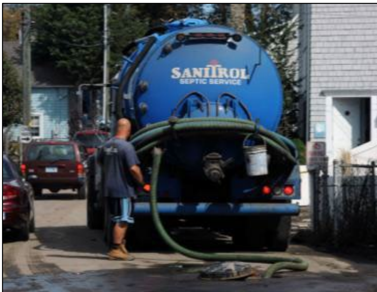
Pumping due to power loss at main lift station, Connecticut Courtesy FEMA
